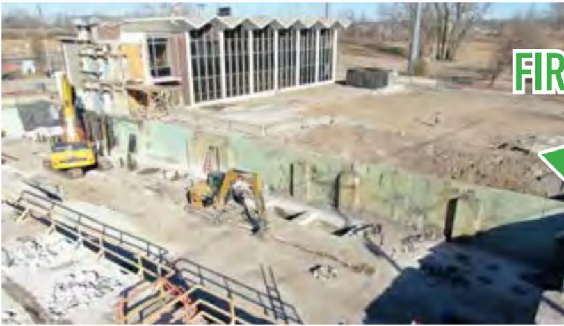
At the beginning of 2022, crews finished demolition work of the former KC Water Blue River Solids Processing Building and incinerator stacks to make room for a new, state-of-the-art building that will utilize the Thermal Hydrolysis Process (THP).
