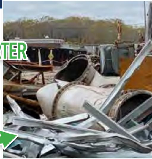
As part of the demolition process, materials were carefully separated and approximately 98 percent of the old building was recycled. A total of 1,600 tons of materials will be reused - that weighs the same as 16 blue whales or 30 African elephants!
