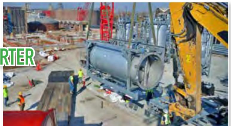
As foundation and basement work continued, the new THP equipment was delivered and installed. This is the biggest upgrade at the Blue River Primary Wastewater Treatment Plant since the plant began operating in the 1960's.
