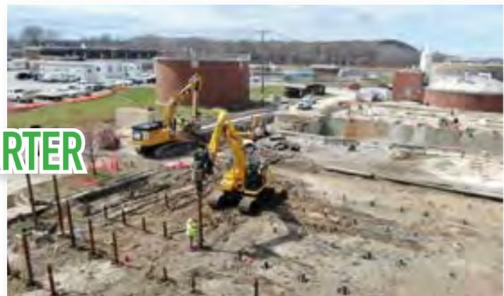
Once the site was cleaned up, it was time to start building the new Biosolids Processing Building from the ground up. Crews installed 246 helical piles to support the Cake Loadout Structure, THP System and the new Biosolids Processing Building.
